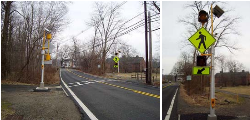
Solar-Powered Crosswalk Warning Device with Buttons at Two Heights
