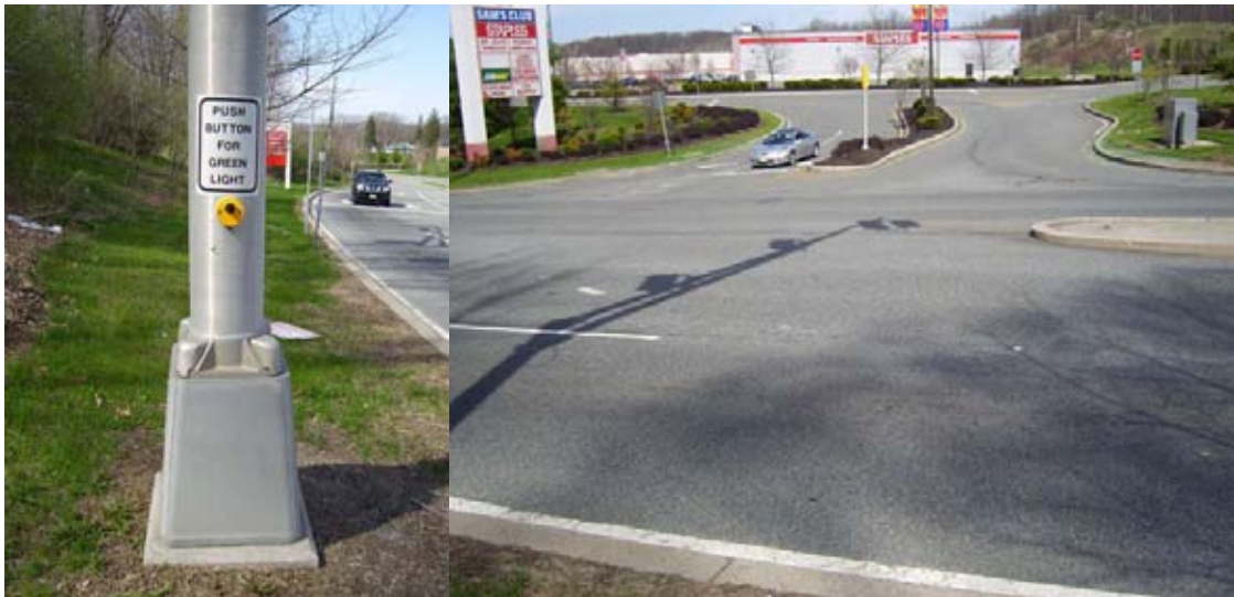
Pedestrian Crossing Button and Lack of Crosswalk Striping on International Drive S.
